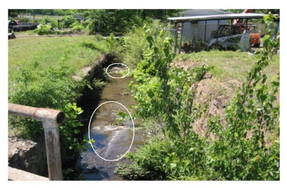
Downstream view of Academy Center Branch from Kerr Street. Channel has natural bottom but walls are made of stacked stone. Dimensions: ~7-ft deep, ~12-ft wide. Note white foam and bubbles on the surface, as well as urban trash.
